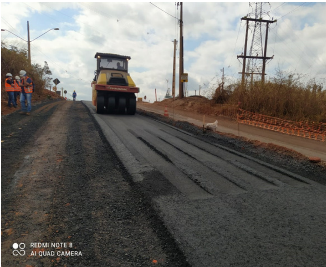
Figure 2: Cauê Experimental Track - Execution Stage
