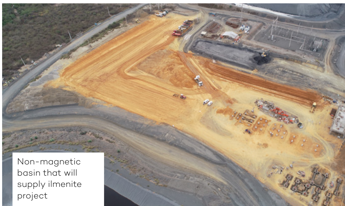
Figure 1: Implementation air view.
