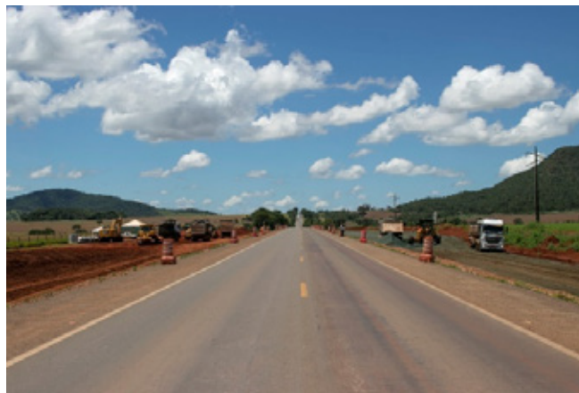
Figure 6: Paving area expansion activities with slag usage at the margin of Concessionaire Highway
