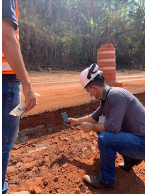
Figure 1: Cauê Experimental Track - Execution Stage
