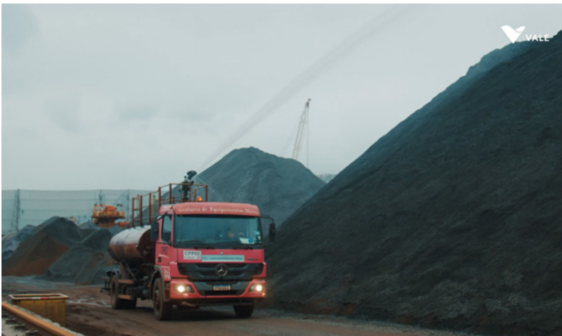
Sustainable Suppressor being applied in Tubarão site (Vitória/ES)
