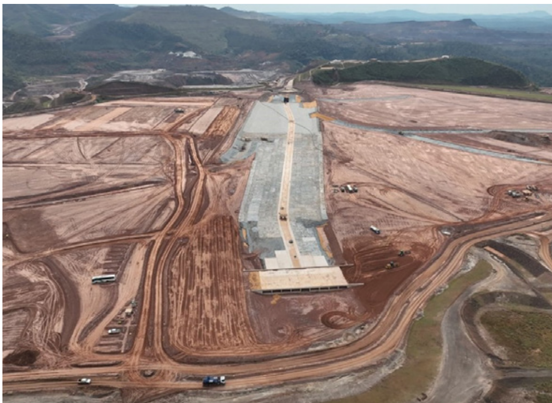
Reservoir reformation with compacted sandy tailings and superficial drainage system implementation.
