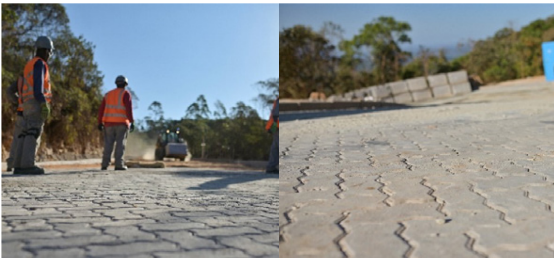
Implementation of blocks made of sandy tailings
