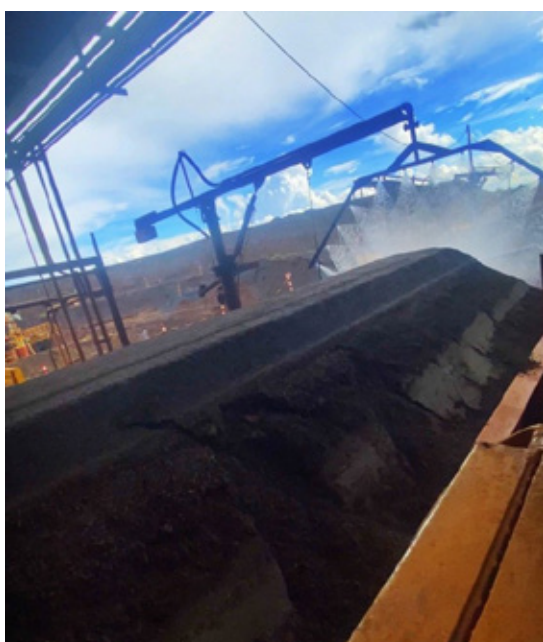
Sustainable Suppressor being applied in iron ore train wagons in Brucutu/MG
