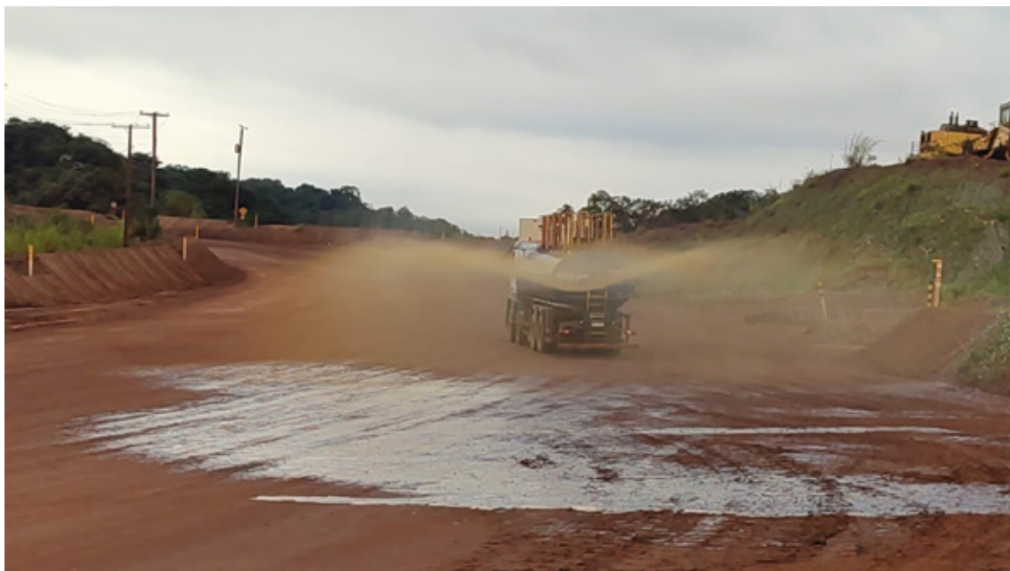
Sustainable Suppressor being applied in unpaved roads in Mariana/MG Complex
