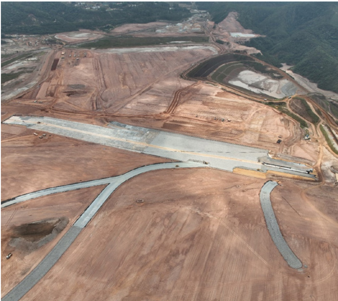
Reservoir reformation with compacted sandy tailings and superficial drainage system implementation.
