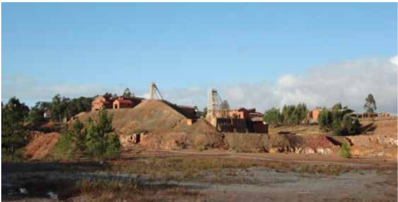
Figure 16: Old industrial unit of the mine that will be rehabilitated for future visits
