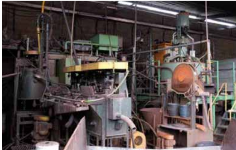
Figure 8 – Adjustable plant used for testing in Gorceix Foundation. [1]
