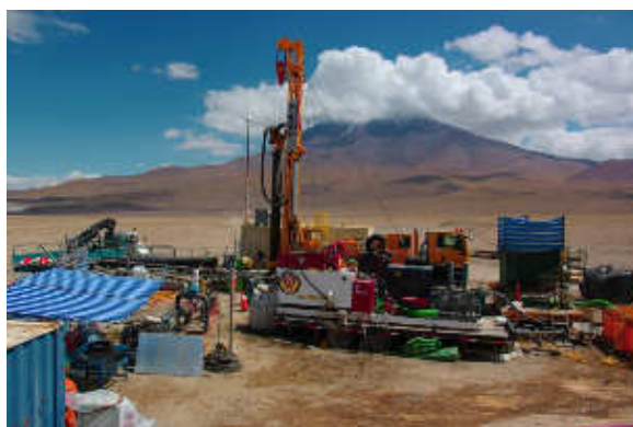
Figure 10 – Large Diameter Well Drilling
