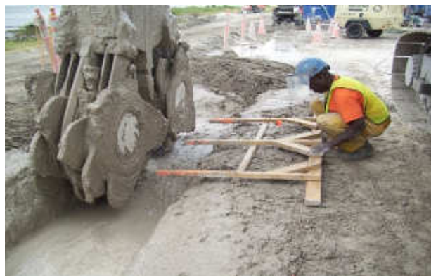
Figure 12 - BAUER BCM 5 CSM Cutter wheel assembly
