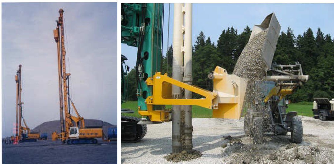
Figure 9 – Installation of gravel columns
