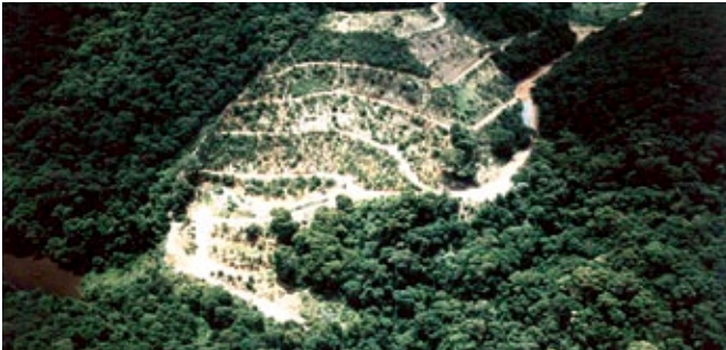
Situation of the waste rock dump A in December 2002.
