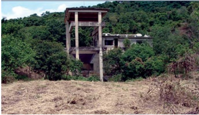
Situation of the primary crushing facilities prior to demolition (2008).
