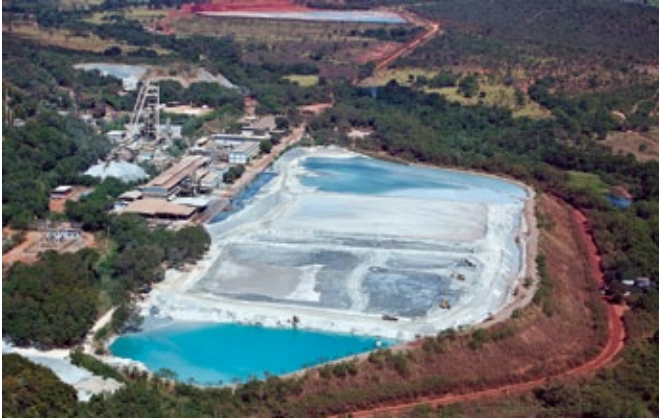
Aerial view of the tailings pond, the industrial facilities and the headframe of the underground mine.
