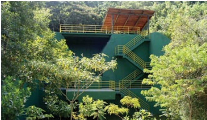
Observatory built in the former primary crushing facilities (2012).
