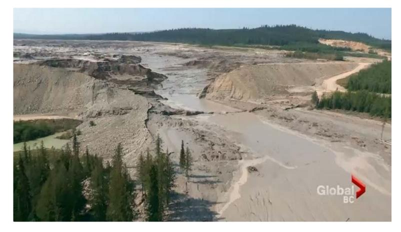
Failure in the foundation of the embankment due to a weak layer that was undetected. The rockfill had very steep downstream slope (1.3H:1V). Had the slope been flattened to 2H:1V, as proposed in the original design, failure would have been avoided.
